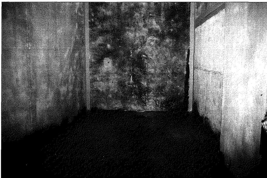
Bare concrete walls form an exercise “yard” at Pelican Bay where prisoners engage in solitary recreation. An opaque roof covers half the yard; the wire screen which covers the other half provides prisoners with their only view of open sky.
